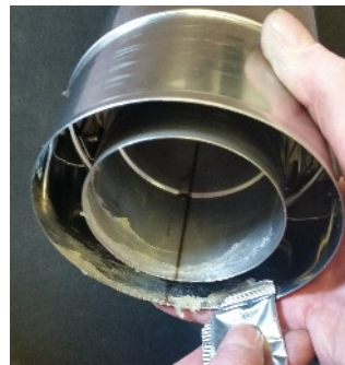
6. APPLY A GENEROUS AMOUNT OF GREASE TO FEMALE SOCKETS TO AVOID DAMAGING SEALS.
