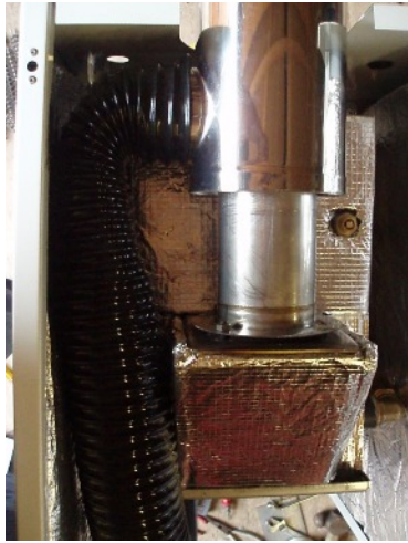
1. LOW LEVEL REAR OUTLET FLUE. KIT PT. NO. FL80LL
