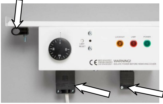
Fire valve sensor retaining clip
