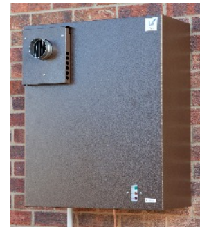
Fit flue terminal
