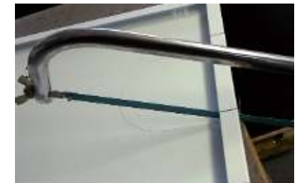
8. HIGH LEVEL FLUE INSTALLATION, CUT MICRO JOINTS, TWIST BLANKING PANEL TO REMOVE. CUT ROCKWOOL INSULATION TO SUIT.
