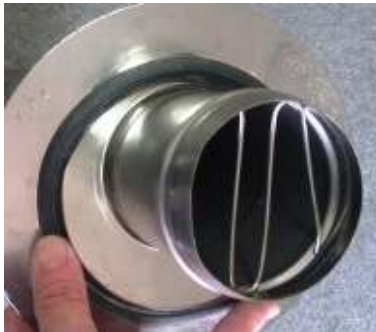
5. FLUE TRIM - APPLY GREASE TO RUBBER SEAL SLIDE TRIM INTO POSITION.
