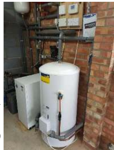
Tuscan 12/19 with 150 ltr. pressurised domestic hot water cylinder. (Replaced a combi boiler)
