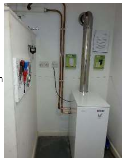
The Sir Max Atkin a converted life boat. Tuscan 12/19 external boiler firing on diesel.
