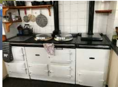
Helmingham Hall, Suffolk. A Tuscan Kitchen model boiler converted to fit in the casing of an Agamatic boiler provides heating and hot water to living quarters.
