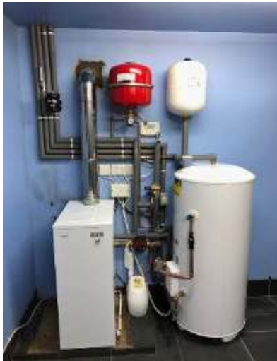
Tuscan 20/25 with 150 ltr. pressurised domestic hot water cylinder. (Replaced a combi boiler)
