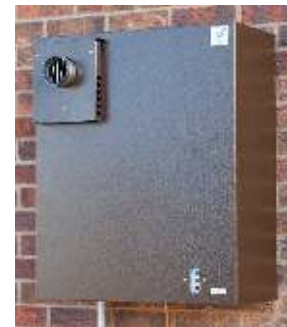
Fit flue terminal
