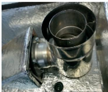
High level & vertical flue connection.
