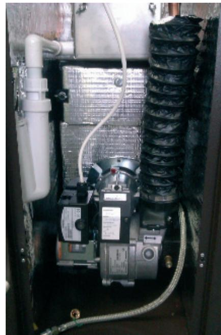
The flexible oil, isolation valve & 10mm compression fitting come pre assembled. Burners are test fired but will need commissioning once installed.
