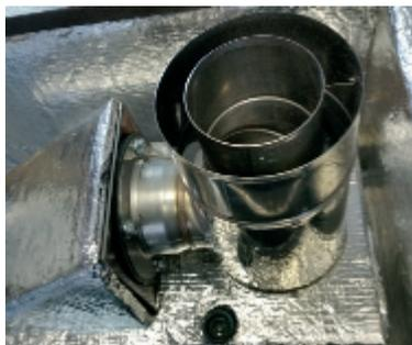
High level & vertical flue connection.
